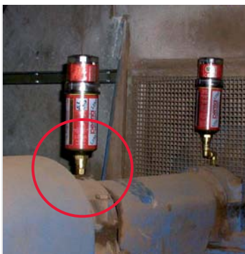
Fan drive shaft lubrication (2 points)
